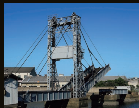
Suehiro Bridge (Nationally designated important cultural asset)
