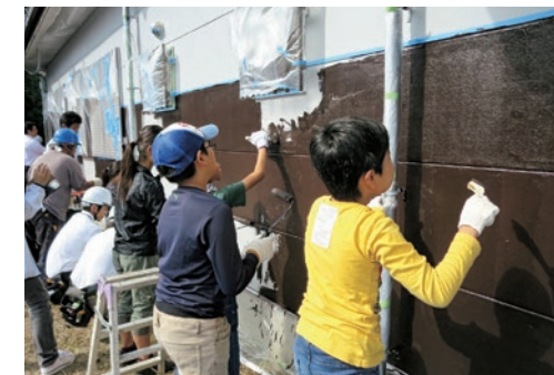
Painting a station building (Hinaga Station)
