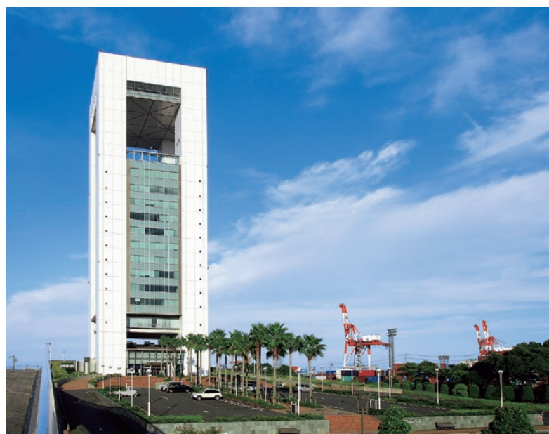
Yokkaichi Port Building
